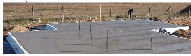
As early as after only several days the foundation is ready, i.e. the underground structures are completed. Izodom slab is an element the exceptionally simple construction of which precludes the possibility of making mistakes. Its monolithic structure is much more stable than the currently designed foundation footings and walls, and the insulation provides a passive standard. We also invite you to participate in free trainings in the company headquarters.
