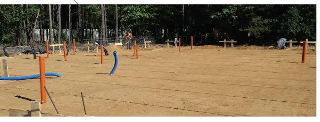
The first stage consists in the removal of the layer of humus and native soil to the depth specified in the documentation. Then one should proceed to the placement of water and drain installations and other utilities. Once this stage has been completed, a filter layer of coarse gravel or key aggregate should be laid on an exposed load-bearing substrate and compacted properly, and then a layer of foil should be spread.
