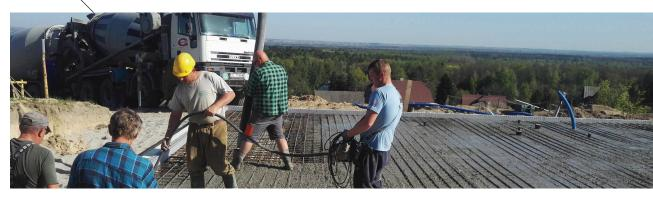
The formwork is filled with concrete of the right grade and texture. Always follow strictly the design and concrete manufacturer's recommendations. This solution allows to obtain a slab without thermal bridges that meets the standards of passive houses.
