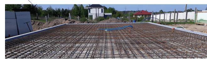
After installation of the slab, the reinforcement is installed in accordance with the documentation. This may be fibre or traditional mesh reinforcement; also, a combination of these two solutions can be applied.
