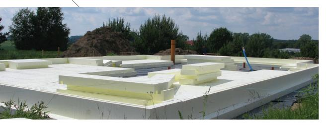
The formwork elements of the ground slab are **cut to size already in the production plant according to the custom design**. On the construction site they are laid in such a way as to obtain a given size and shape of the slabs. The kerbs and corners are connected using dovetail joints. Next, the **bottom elements are laid** – they are joined with kerbs using hook bolt locks. At the end, they are complemented with cut-to-size elements.
